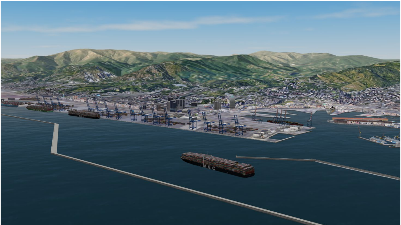
Figure 4.10: Arrival of ULCS in laden conditions – Run 21
